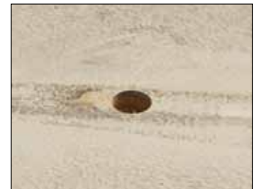
Dark, wet core spewed out of some of the holes, left. Other holes had light-colored, dry and healthy core.
