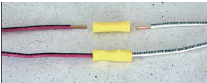
Use crimp-on connectors to attach the wiring for the light.
