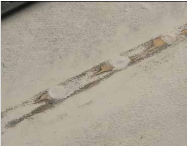
The enlarged holes filled with epoxy. More sanding will smooth them.
