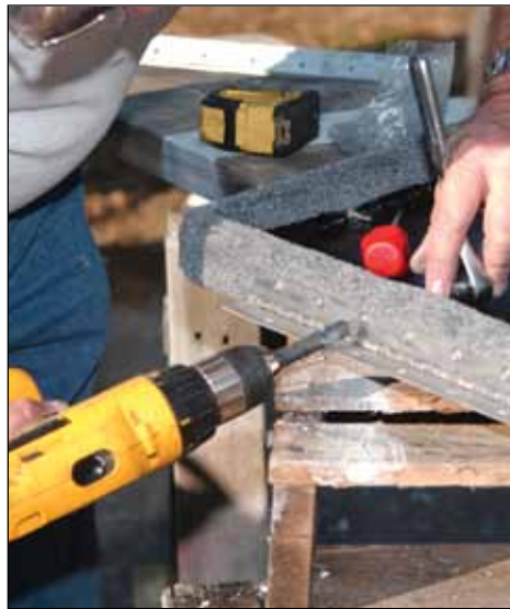
Replace hinges and latches using new stainless hardware.
