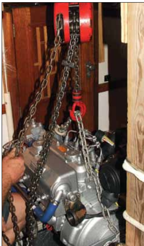
A chain hoist was used to lower the new motor into the engine room.
